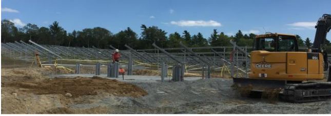
Figure 4. Photo of anchors being installed in preparation for solar racking installation at Dartmouth Farms Solar. Photo courtesy of Nexamp LLC.
