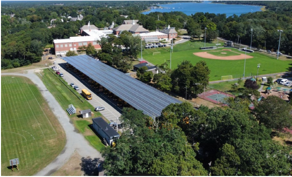
Nauset Middle School Solar PV with BESS
